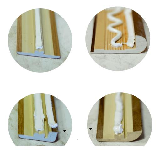
The Overlap Reducer and Square Nose Can either have one or two strips of glue. Both options are shown above.
